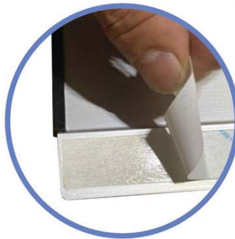
Remove and install double-sided sticker film
